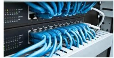
Imagen 72: Switch. Nota. ms.gonzalez (2012), redstelematicas (<https://redstelematicas.com/tipos-de-switches/>)
